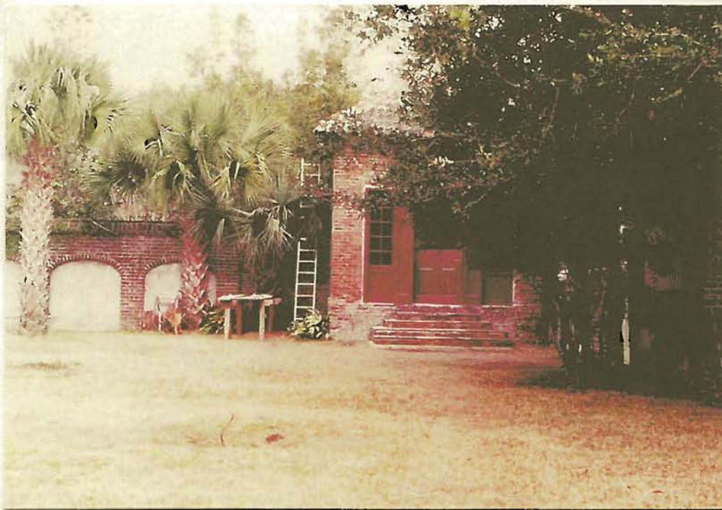
221 Figure 69. View of Brewton privy and enclosure
