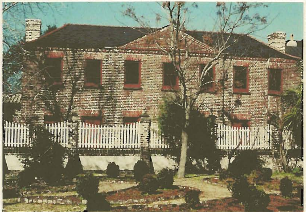
Figure 10. View of the antebellum quarters building
